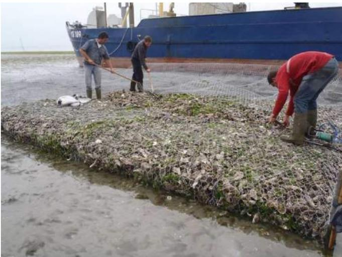
Figure 2.4 Artificial oyster reef - an example of Building with Nature to create new a habitat and mitigate wave height (source: EcoShape).
